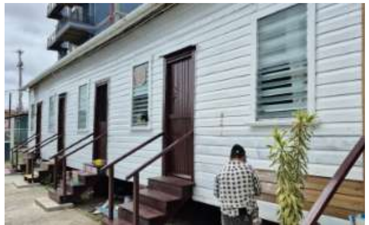
An image showing completed works at the Care Home.
